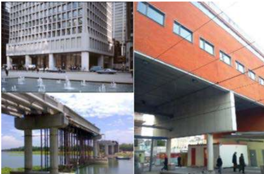
Figure 1. Application areas of reinforced concrete deep beams
