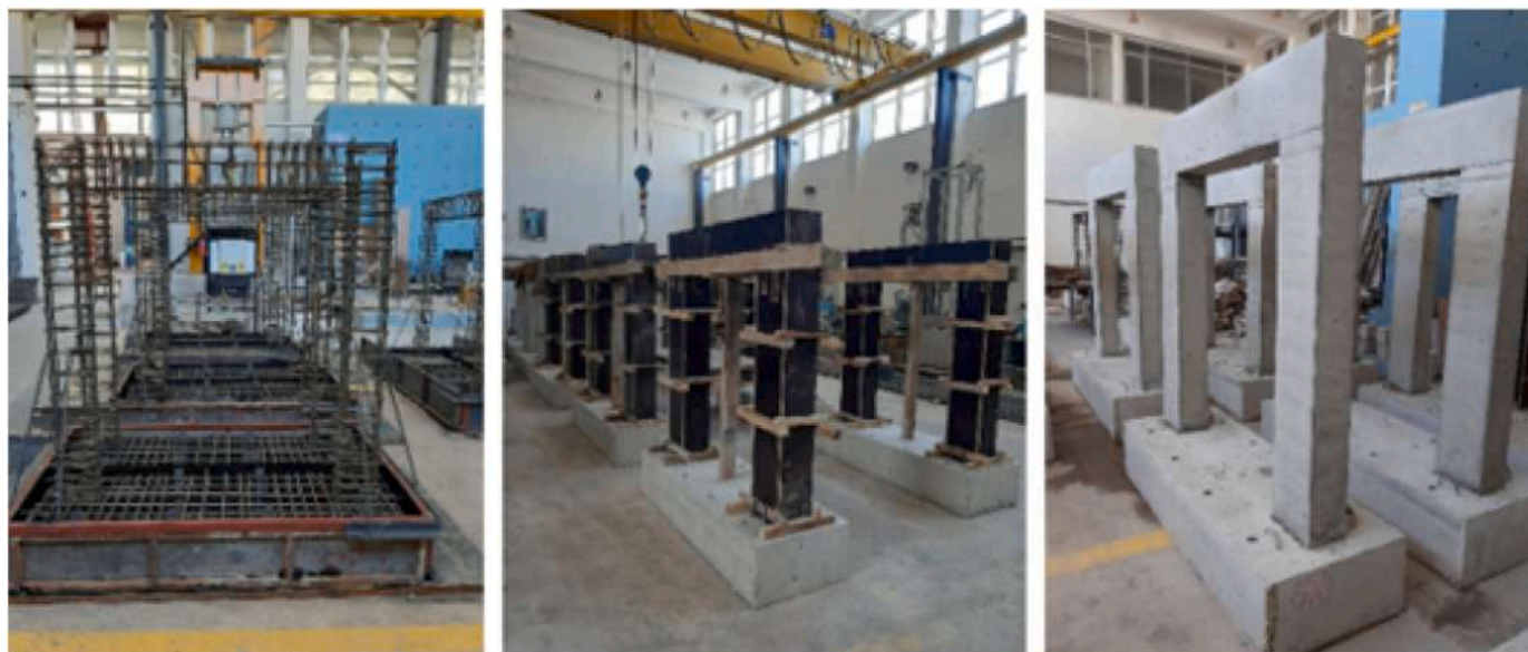
Fig. 4. Production of the reinforced concrete frame test specimens.
